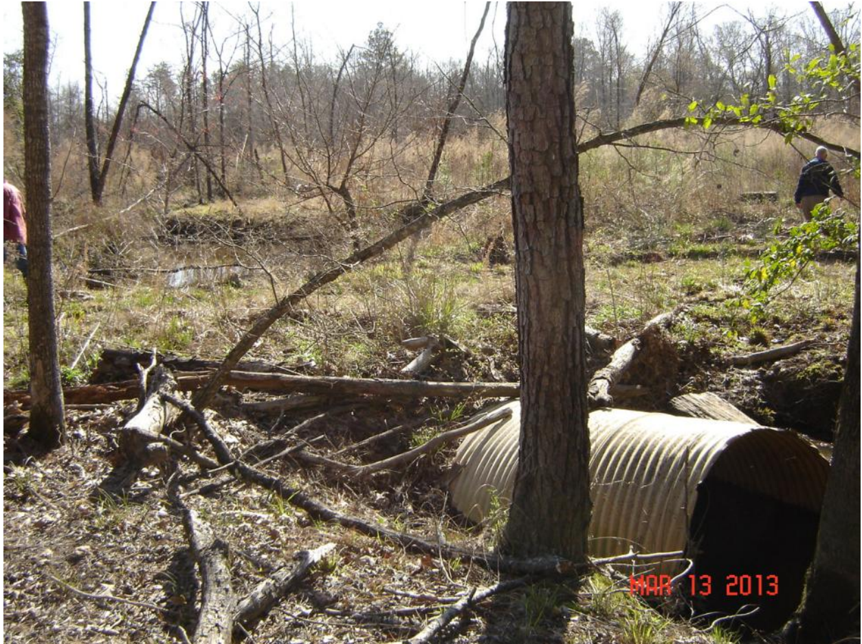
Road crossing on Little Bayou de Loutre that will be replaced or removed, 3/13/2013
